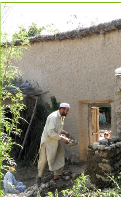
Returnee repairing his damaged house
