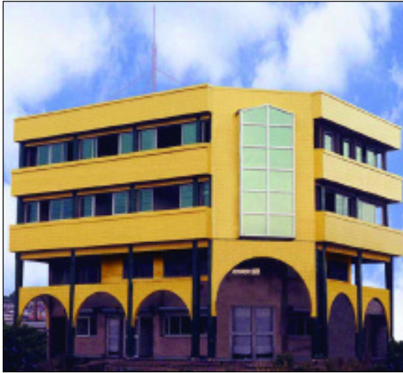
Above: ICT Training, Kigali, Rwanda
